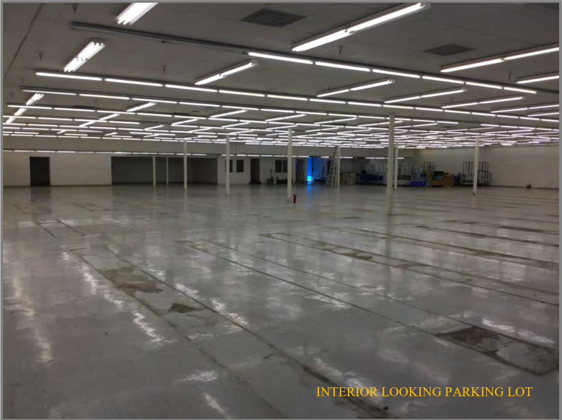
INTERIOR LOOKING TOWARD F STREET
